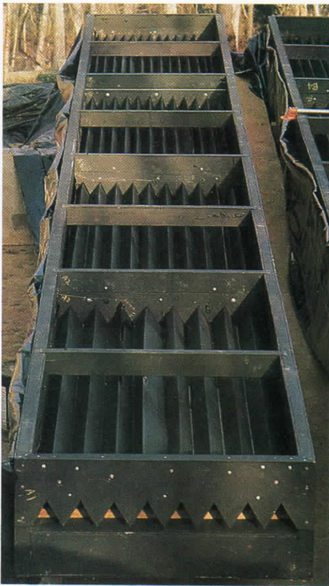
Combining active and passive. Above right, protected by temporary covers, Levine's active collectors are hoisted into position on the south face of the house. Each of the seven active collectors, above, is 32 ft. long and was built on the ground from standard materials. Levine glazed the space between active collectors (drawing, right), creating what he calls sundows for passive-solar gain.
