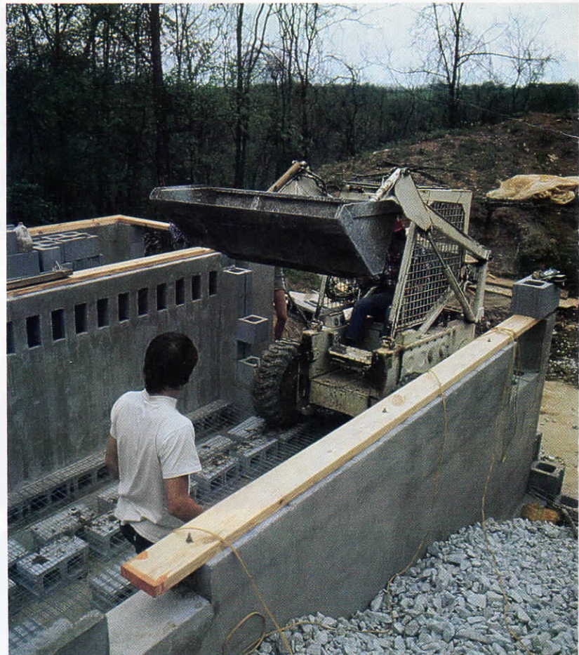
Rock storage. Eighty-five tons of mass in three separate rock bins can be heated individually or together by the forced-air system (drawing, left). Above, the vented mesh, shown here being covered by a load of crushed limestone, allows air to travel down through one rock bin and up through the next for maximum heat transfer.
